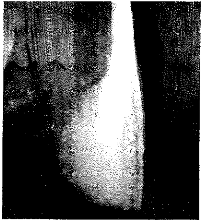
(b) Frost accumulations at rafter bridge joists due to air leakage
