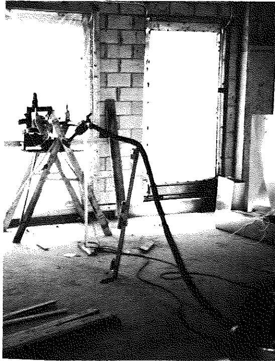
Figure 4a. Component depressurization and pressurization test for air leakage control and specification requirements
